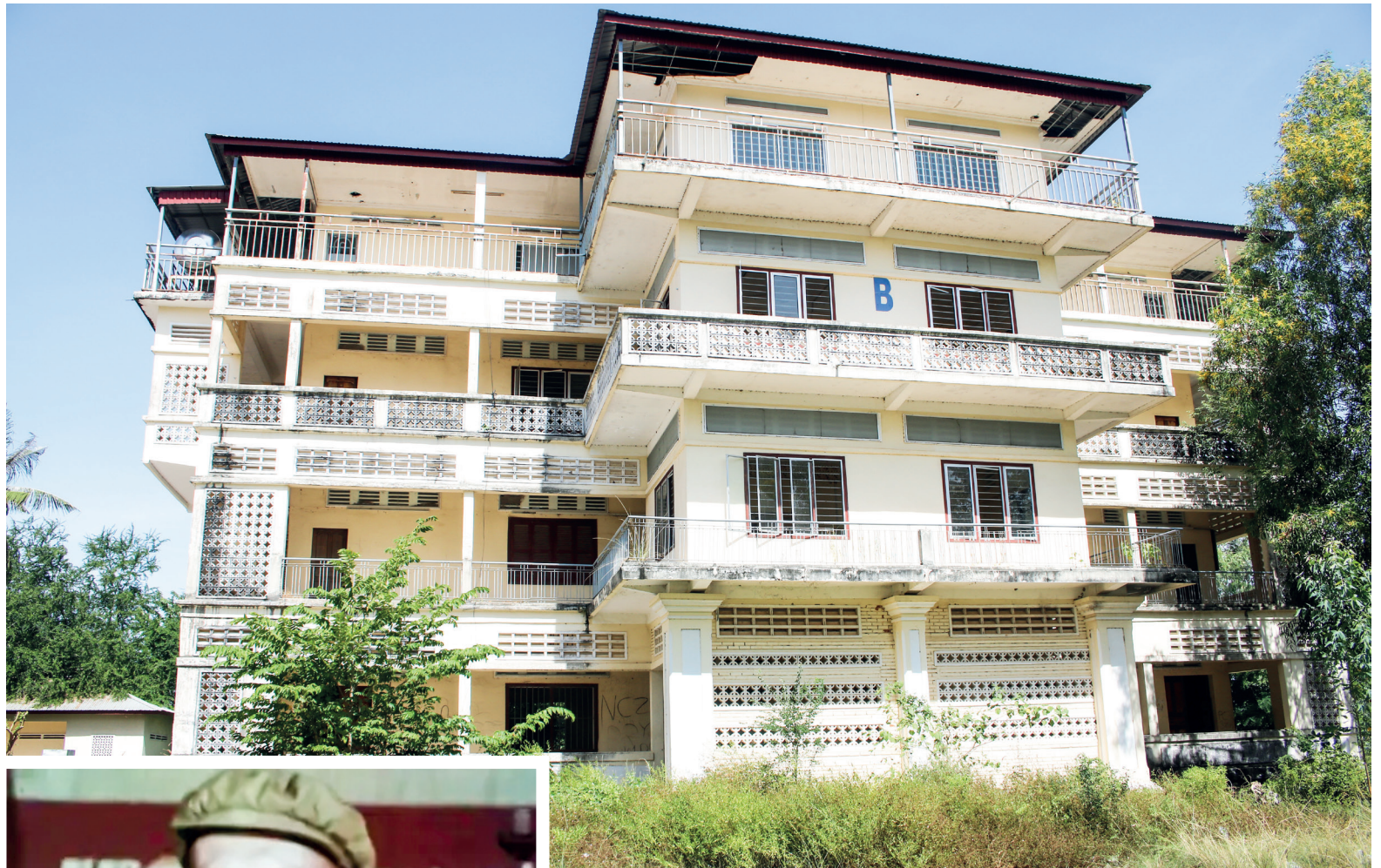
The former lakeside home of Takeo province's most notorious son. Men Kiri
