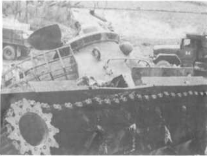
DISABLED M48 OF THE SOUTH VIETNAMESE 20TH TANK REGIMENT. Road wheels received hit from rocket near My Chanh River.
